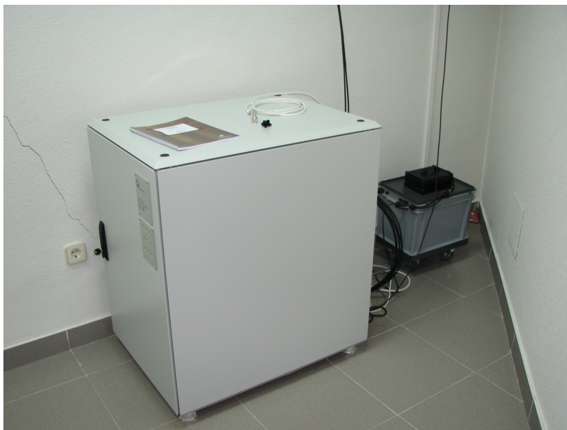
Figure 1: EFOS Maser S/N 66 in its room. Battery at the bottom.
