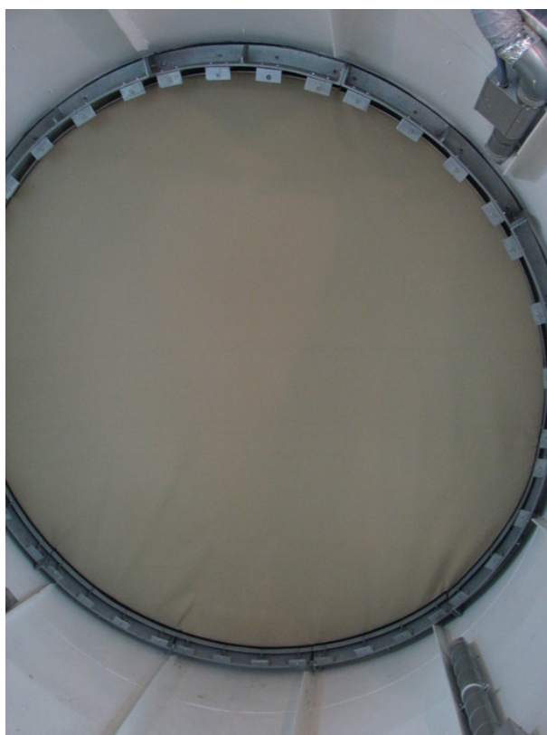
Figure 3: Picture of the old membrane with the heavy iron support structures forming a circumference.
